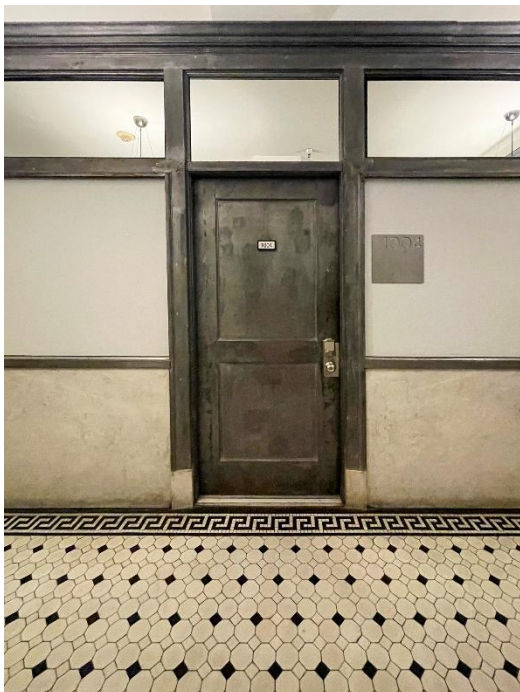
Photo 28 Entry to individual unit, showing zinc-clad door and mirrored former transom windows. View toward door, camera facing south.
